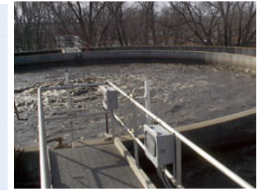
Waste water treatment.
